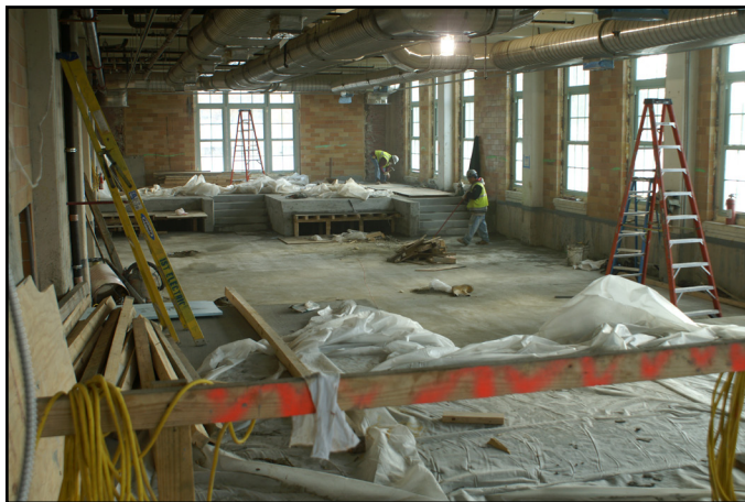
After: current view of new tank platform
