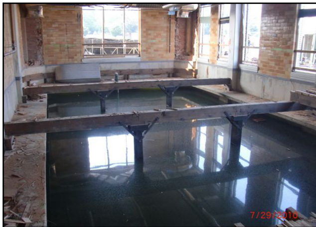
Before: old floor torn up to reveal creek water
